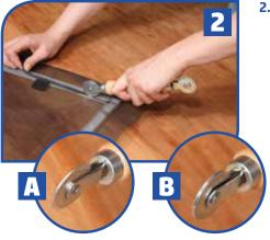
2. A: For aluminum screen: use the convex end of screen tool to gently roll screening into the frame groove to crimp screening.
