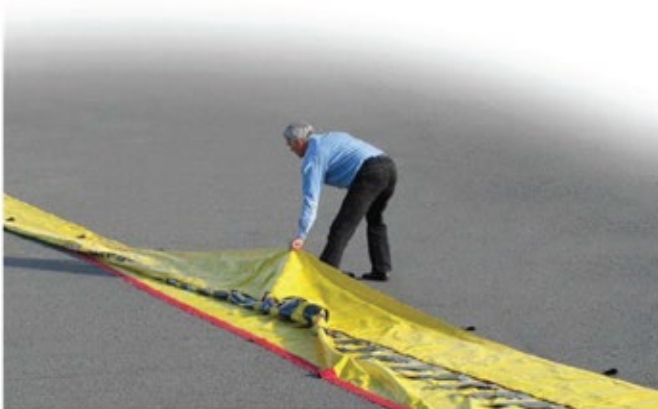
A - Completely unfold the Water-Gate.
